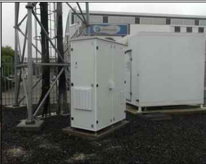
SITE VIEW (INSIDE)
